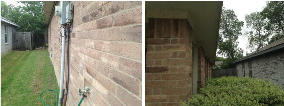
Pictures 1 and 2: Brickline deflection along the left and right sides.
