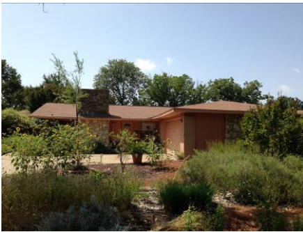
Photo 1: General view of the front of the home.
