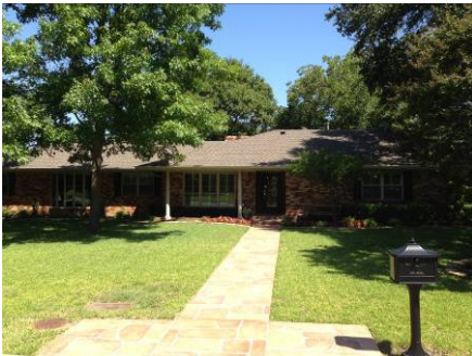
Photo 1: General view of the front of the home.
