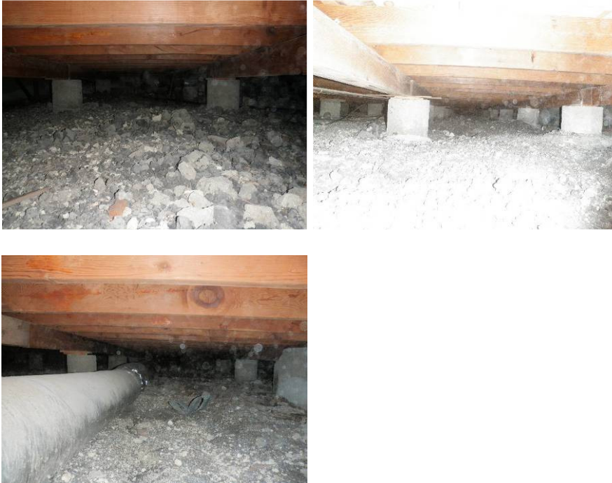
Photos 11 - 13: Views beneath the home.
